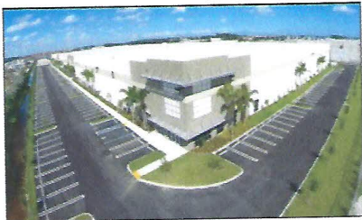
Airport North Logistics Park Phase One
